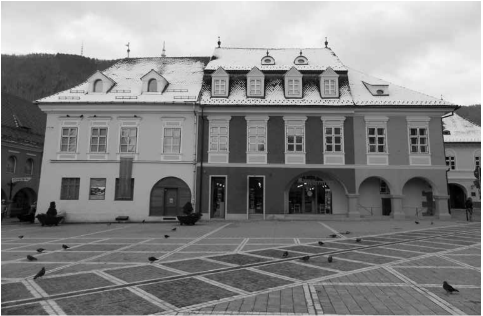
FIG. 1. The ensemble of the three houses on the former Short Row in Braşov, today no. 15–16 Town Hall Square, after restoration.
